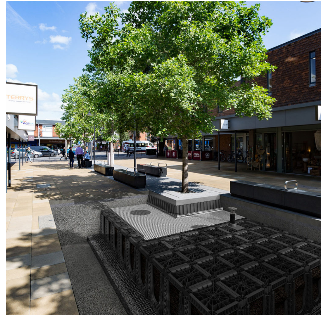
GreenBlue Urban Soil Cell Pavement System Install
