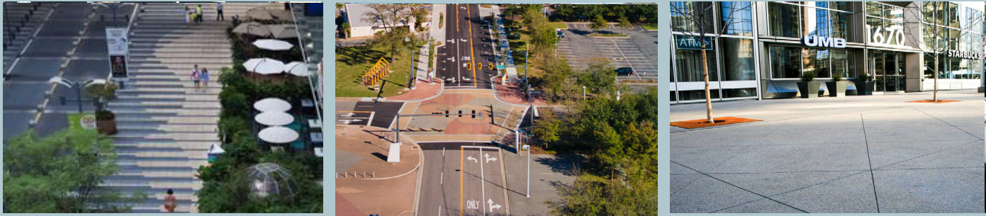
Sawcut concrete, with clean lines are one idea to replace a portion of existing paver areas. This will ease maintenance efforts with the ability to pressure wash as needed. Accent pavers could be strategically located for aesthetic interest in amenity areas and to help delineate right-of-way lines. Pavers could be installed within intersections and/or within crosswalks, especially in key areas such as those within the entertainment zones.
