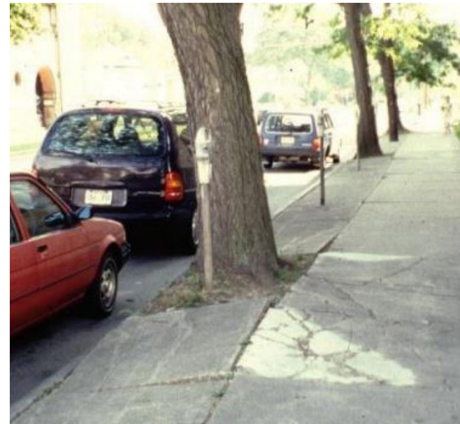
Trees Planted in Limited Soil Volumes Struggle to Survive and Often Damage Adjacent Sidewalks
