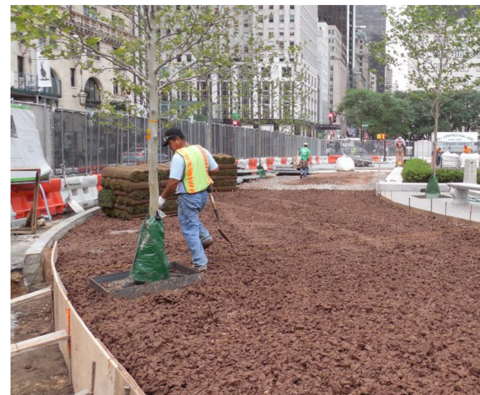
Structural Soil Installation
